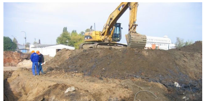
Excavation of contaminated soil
