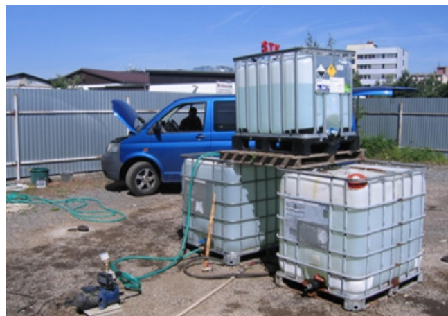
Pilot test of persulfate application within the area of OZT – Toužim
