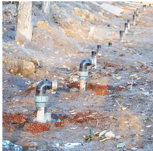
ISCR PRB boreholes after installation
