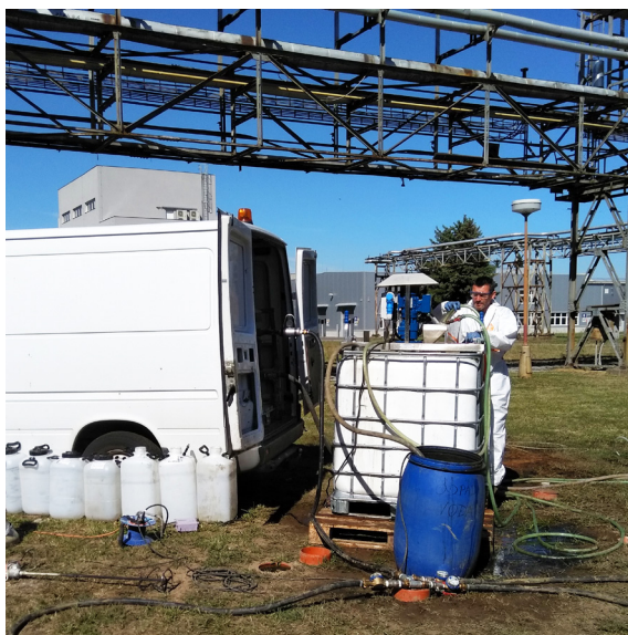
High pressure injection of sulphidized nanoscale ZVI into injection wells
