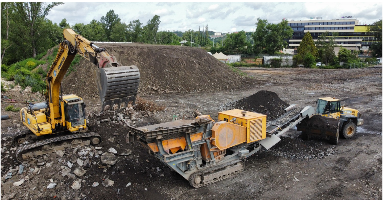
Processing construction waste on a mobile waste crusher
