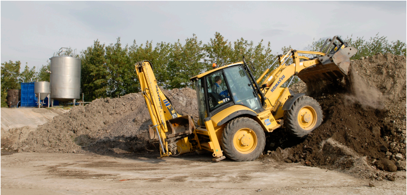
Aeration of soil on the bioremediation platform
